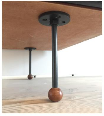
Using a suitable wrench loosen the counter nut at the top of the leg.
